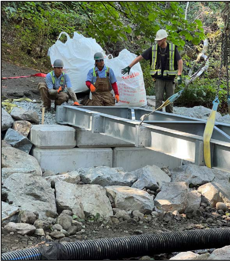
Placing the frame precisely
