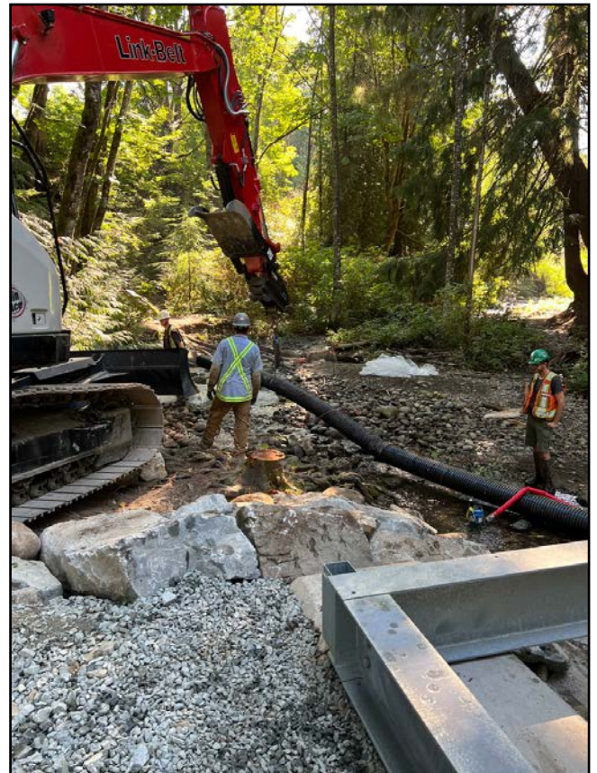
Removing the water diversion pipe
