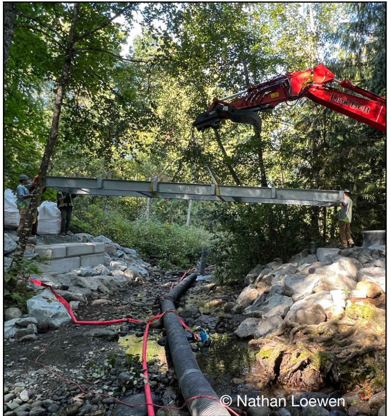
Lowering the frame onto the abutments
