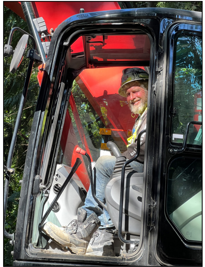
Erv, the expert excavator operator
