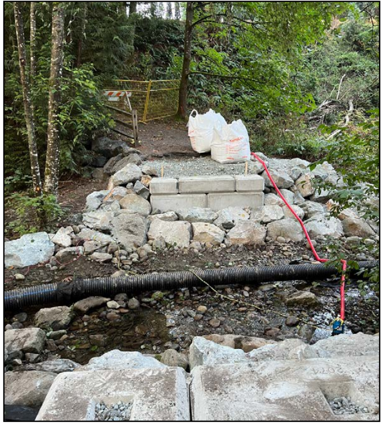
The abutments and riprap are ready
