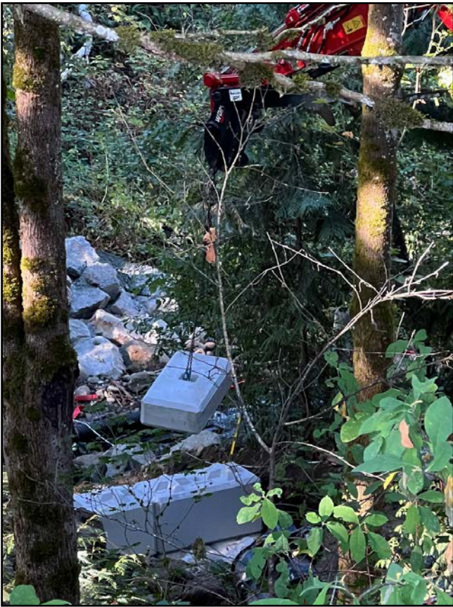
Lowering a cap block into place
