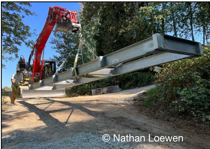
Delivering the steel bridge frame
